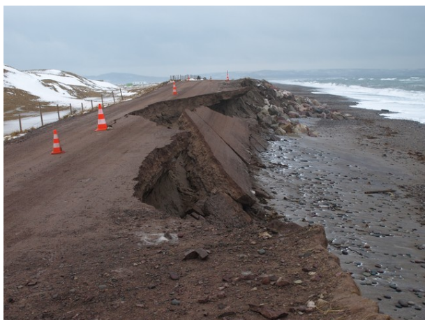
Route des Buttereaux PK18, le 21/01/2009
