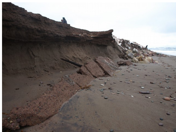
Route des Buttereaux PK18, le 21/01/2009
